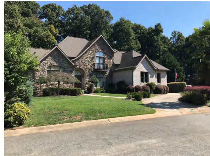
Left of Subject Property
