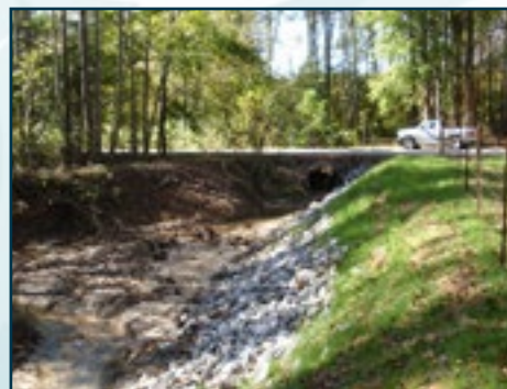
Streambank stabilization
