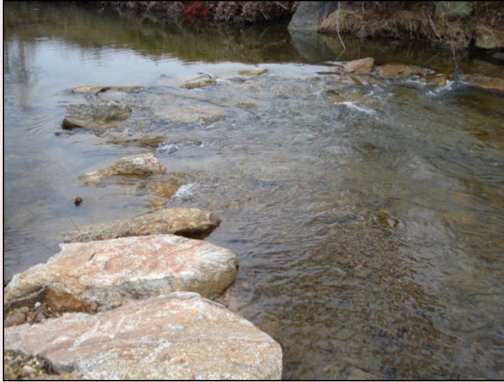
Rock cross vanes, like this one on the Middle Saluda River provide critical habitat for native trout
