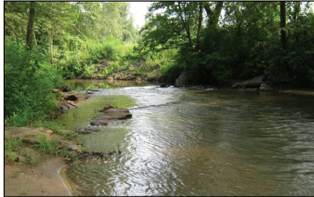
J hook in the Middle Saluda trout habitat project. J hooks allow fishermen to walk to the middle of the stream, provides trout habitat, and diverts the water from eroding river banks
