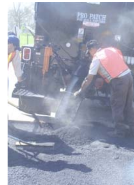
Road Crews Working
