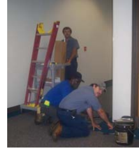
Carpet Repair at County Square
