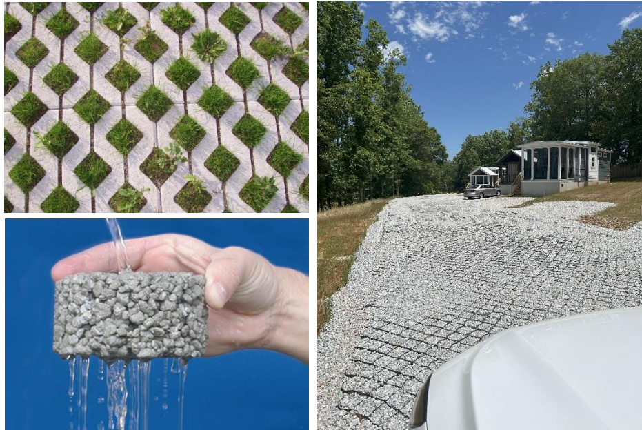
Figure 33 - Examples of pervious pavement including open cell paver stones with soil and grass infill, permeable concrete, and geogrid filled with stone
