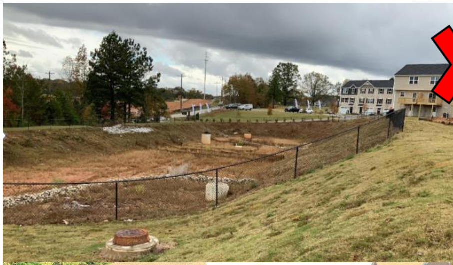
Figure 26 - Chain link fencing provides a needed safety barrier due to steep slopes, but creates separation rather than connection to the stormwater feature
