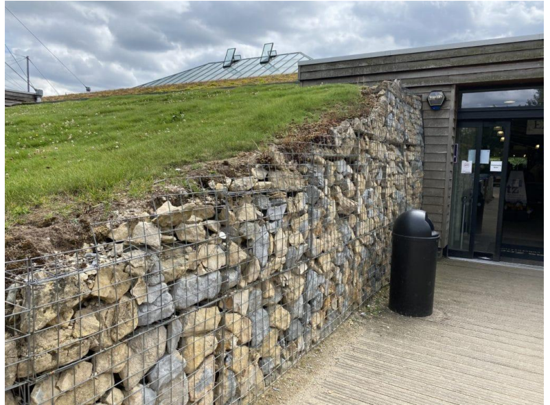
Figure 23 - Gabion basket retaining walls are striking alternatives to traditional retaining walls (Gabion Basket, n.d.)
