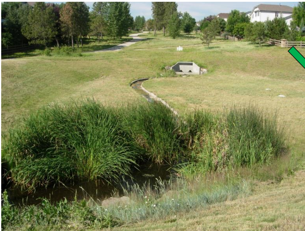
Figure 16 - A dry pond with a low flow channel, partially vegetated (City of Greeley, CO, n.d.)
