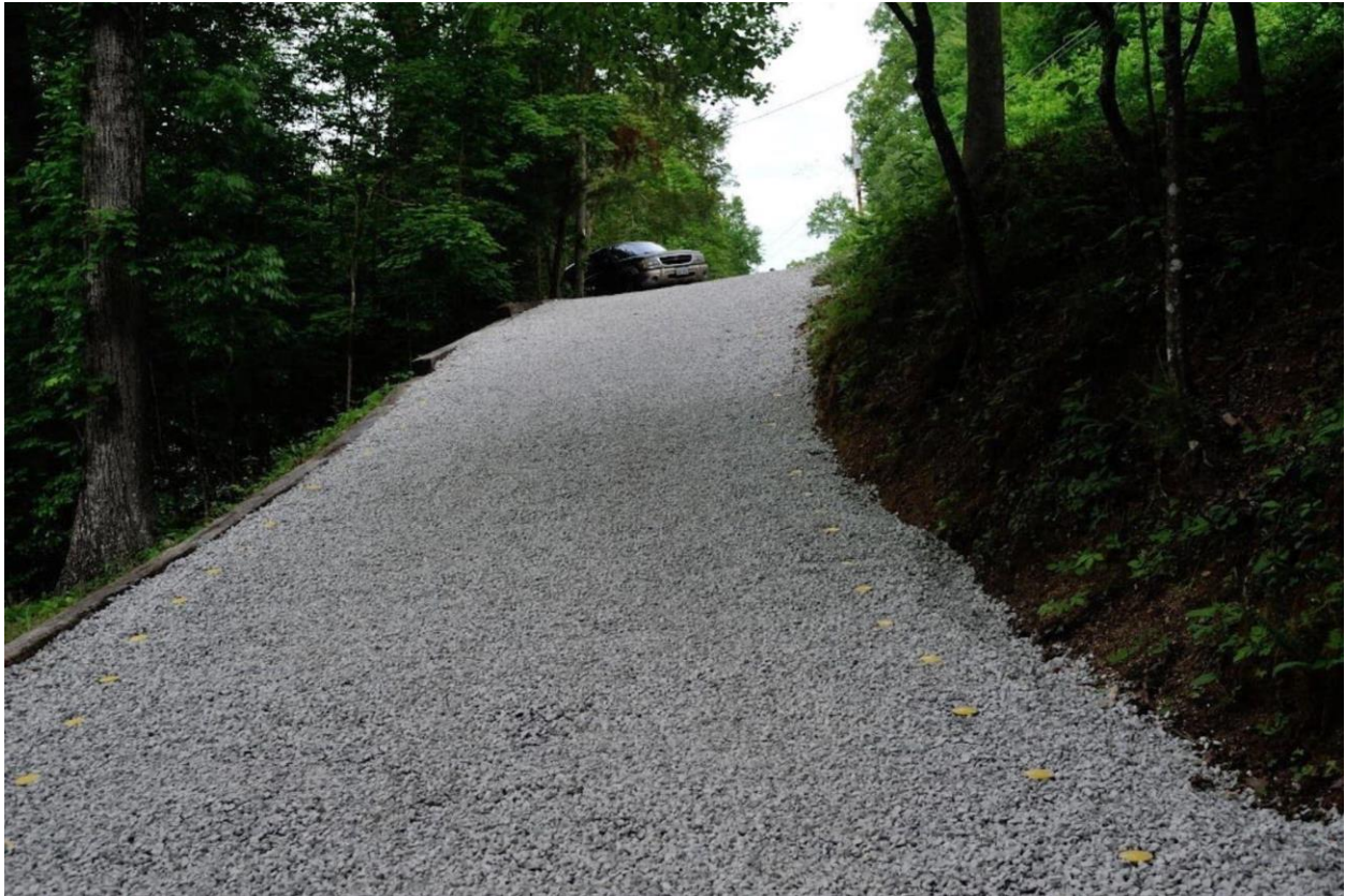
Figure 42 - Pervious pavement surfaces infiltrate water to reduce flows down sloped areas (TrueGrid, n.d.)
