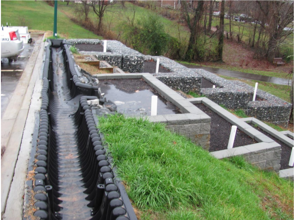
Figure 40 - Bioretention with grade control structures on a steep slope (HydroCycle Engineering, PC, n.d.)
