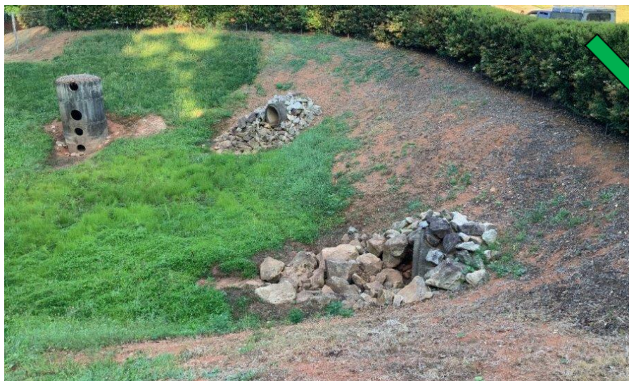
Figure 27 - Vegetative barrier around the top of the dry pond embankment provides a natural option when pond barriers are required for safety
