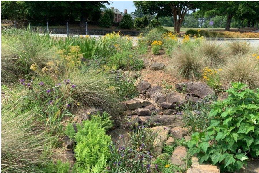
Figure 35 - Enhanced dry swale in Greenville County featuring natural stone and vegetation
