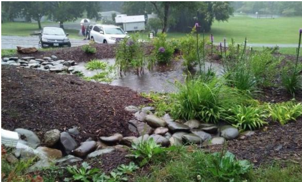
Figure 31 - Rain Garden functioning for retention and later infiltration and filtering (VASWCD, 2024)
