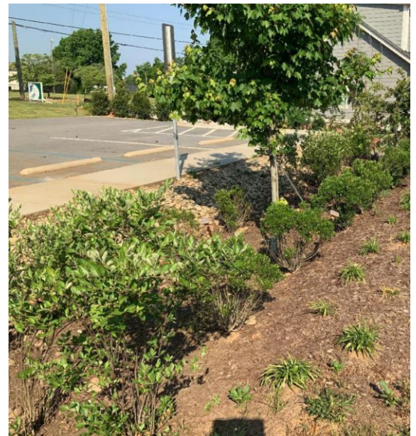
Figure 24 - Left: Roadway and sidewalk runoff enters a bioretention basin through curb cuts (Portland, 2024). Right: Bioretention installed along a parking lot receives runoff as sheet flow (Greenville, SC).
