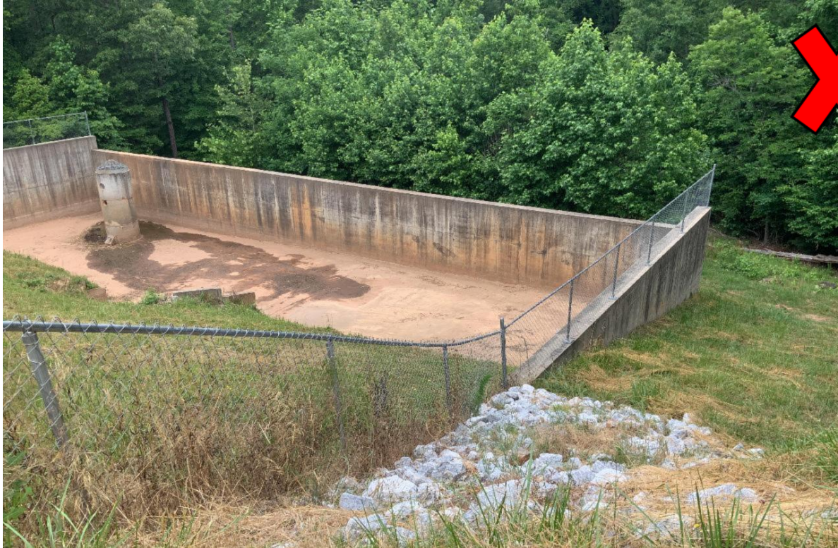
Figure 17 - This dry detention pond features concrete walls and a chain link fence, providing function with no attempt at a natural or aesthetically appealing form
