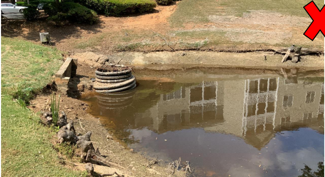
Figure 8 - A lack of vegetation can lead to erosion and poor pond performance
