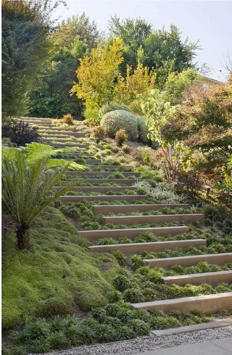
Figure 44 - Terracing of vegetated filter strips can create flow paths with gentle slope to filter water and improve site aesthetics (Risedorph, 2016)
