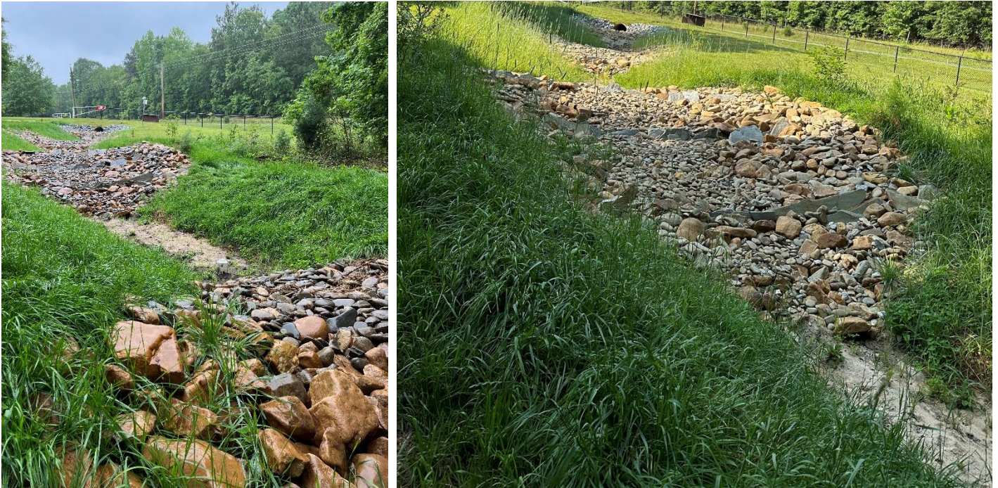
Figure 43 - A regenerative stormwater conveyance in Greenville County provides engineered channel stability while visually resembling a natural streambed
