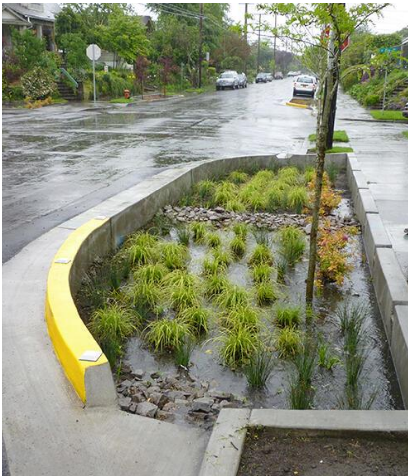
Figure 24 - Left: Roadway and sidewalk runoff enters a bioretention basin through curb cuts (Portland, 2024). Right: Bioretention installed along a parking lot receives runoff as sheet flow (Greenville, SC).
