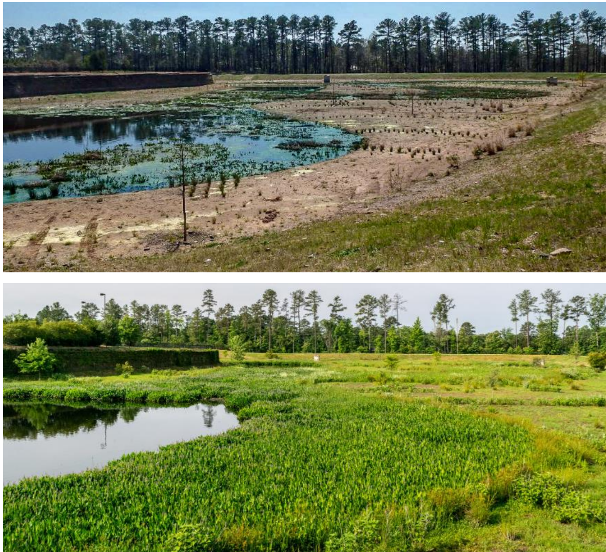
Figure 11 - Monitoring is critical during the years following planting ensure species thrive as designed. Above: initial planting of wetland vegetation. Below: Establishment of vegetation after three years. (Dragonfly Pond Works, 2024)
