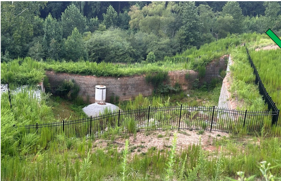
Figure 18 - This dry detention pond utilizes gabion baskets of stone and vegetation to present an engineered structure with features that mimic nature
