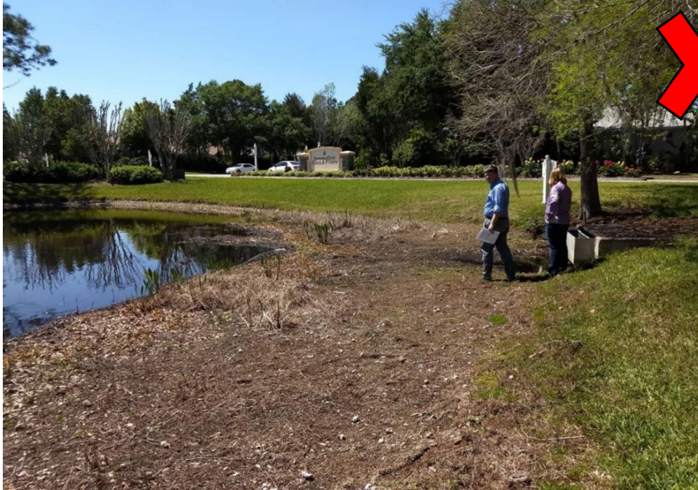
Figure 6 - Ponds with sod to the water line often see severe bank erosion and sediment deposition (Iannone, 2019)
