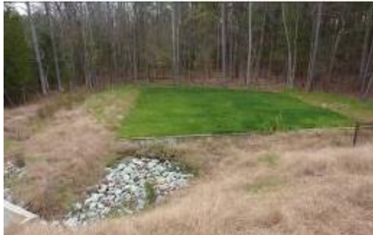
Figure 37 - Above: VFS and level spreader during installation and prior to establishment of vegetation. Left: An established VFS with a well-maintained stand of turfgrass.
