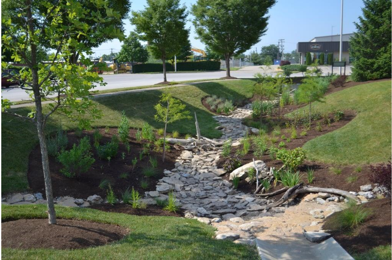
Figure 41 - Rain gardens can be designed to slow and treat runoff flows at the bottom of slopes (Stever, 2016)
