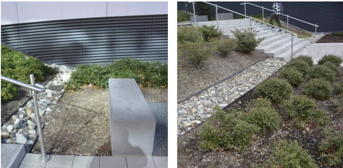
Figure 45 - Stone trench level spreaders installed at the toe of slope to intercept concentrated flow and create sheet flow conditions through areas with engineered filter media and vegetation
