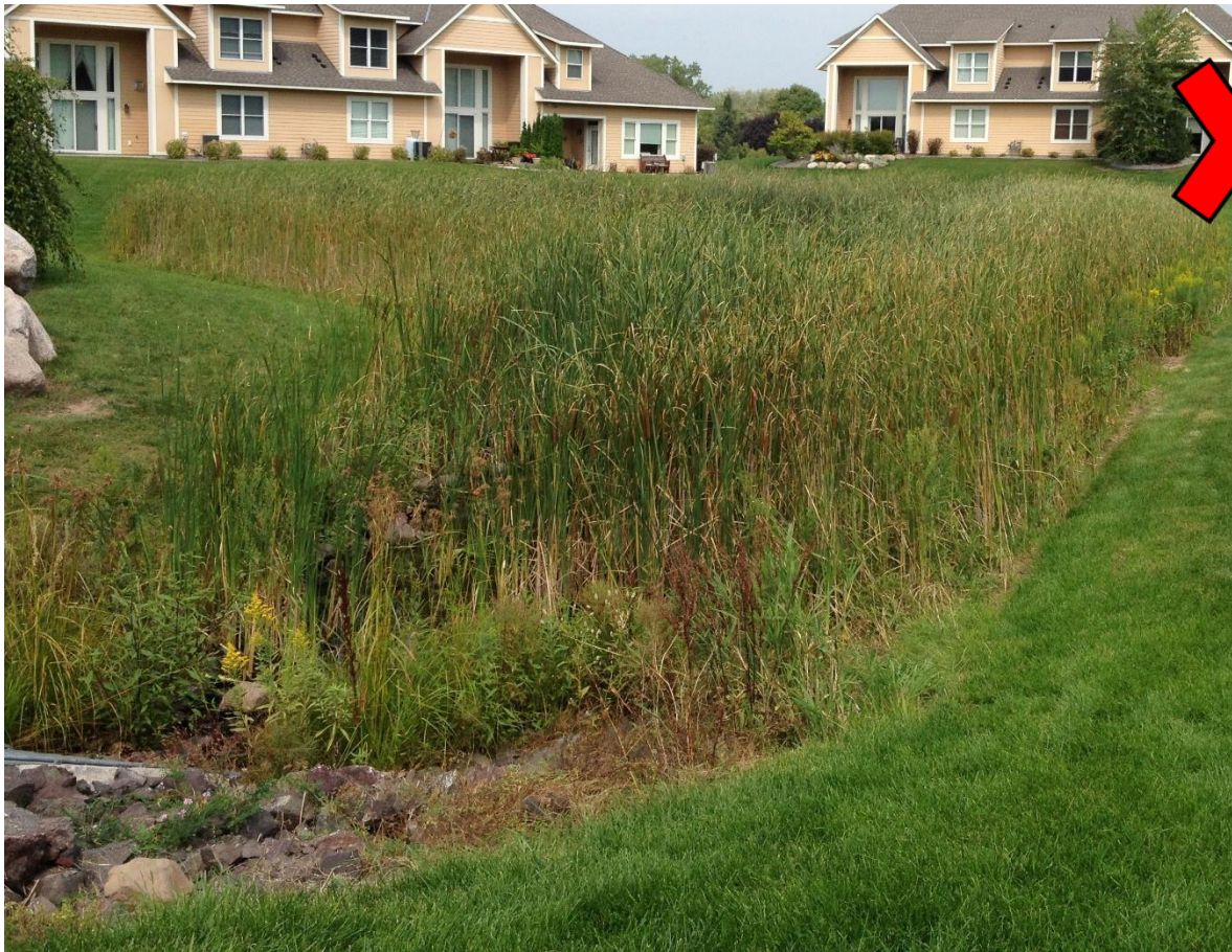
Figure 12 - Invasive cattails and other vegetation have taken over this stormwater wetland (Transform Your Wetland with Invasive Cattail Removal!, 2022)
