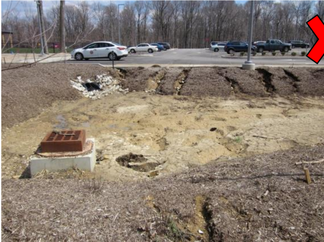
Figure 15 - Lack of vegetation will lead to significant erosion and basin failure (Penna, n.d.)
