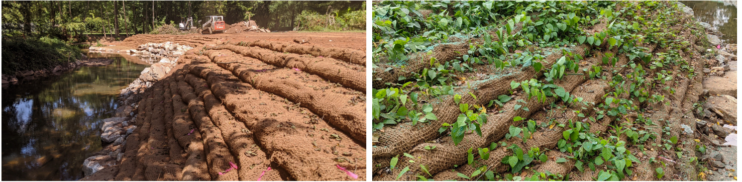
Figure 6. Soil lifts immediately following construction (left) and Japanese knotweed invasion of the soil lifts (right).
