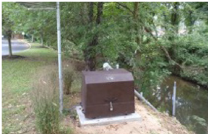
Figure 5. Greenville County monitoring station at Mills Avenue.
